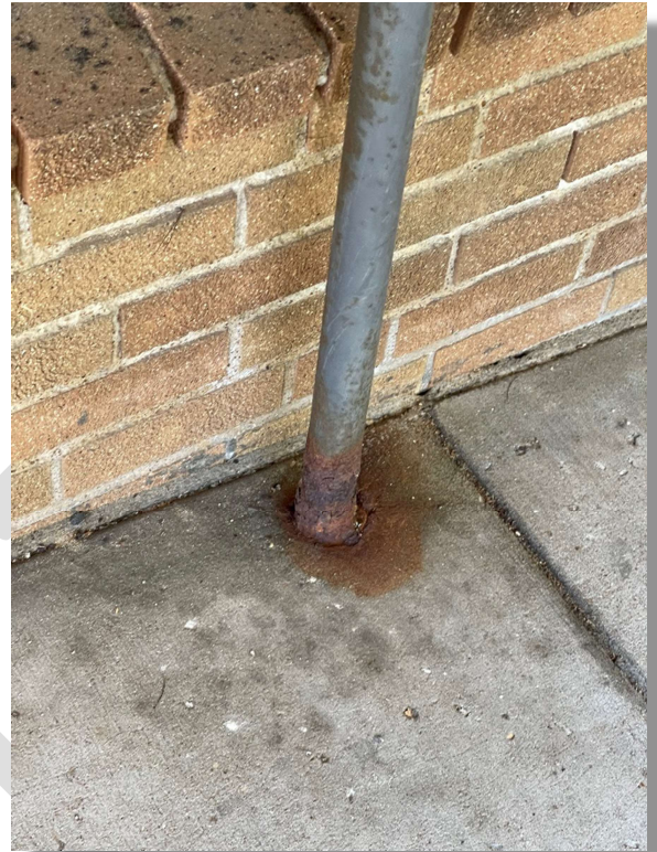
Many of the guard rails / handrails are rusting through and are not properly anchored
