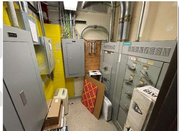
Electrical panels and switch gear is being blocked by storage items resulting in code violations.
