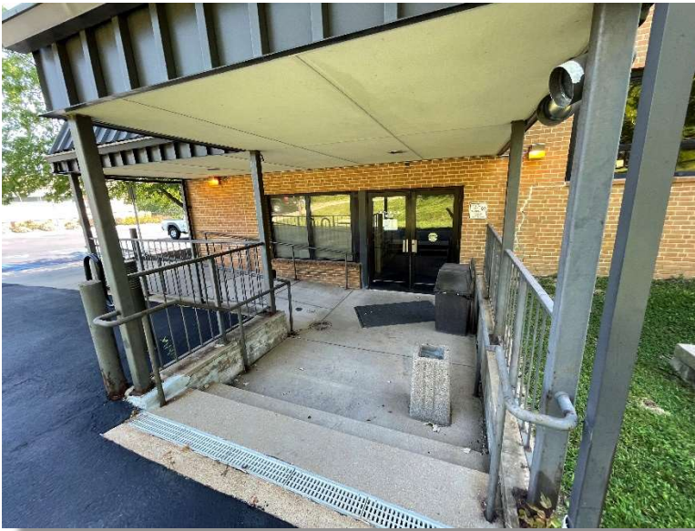
Existing Entry into Community Room – Despite drain at top of step and area drain at landing, entry doors are subject to flooding should area drain gets clogged or covered.
