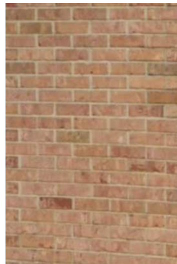
EXTERIOR BRICK AT PLAZA
