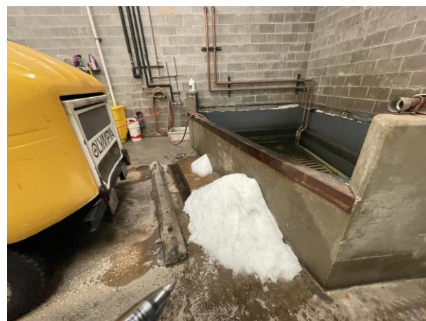
Photo 4 – Existing snow melt pit and coil
