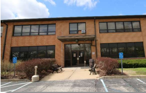
Exterior of East Entrance
