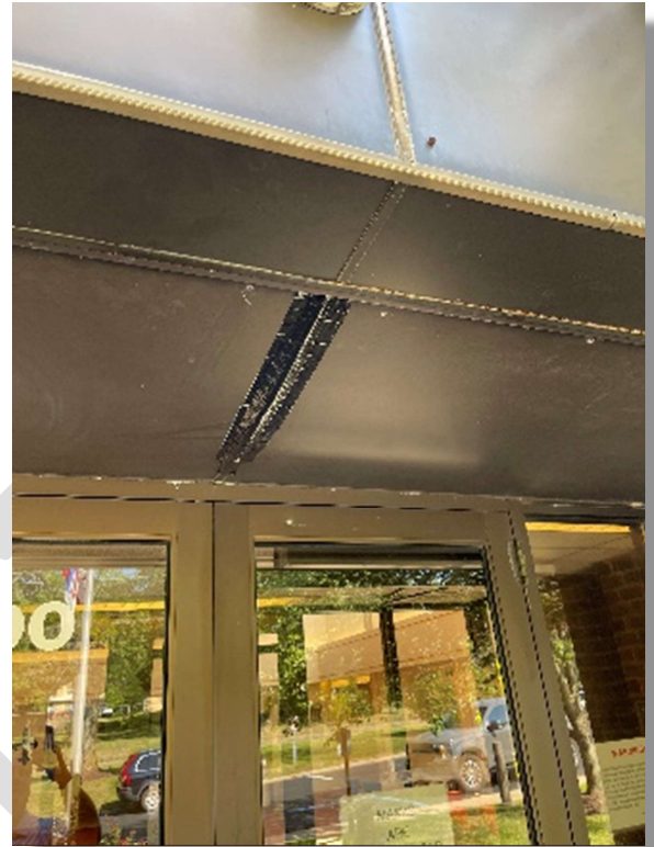
Entrance Canopy seam repaired with black duct tape at center of canopy over Main Entry Doors.
