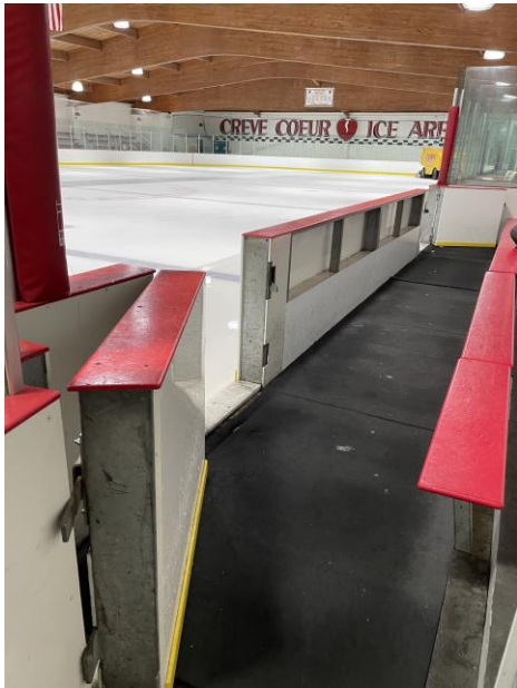
Photo 7 – Existing dasher board system
