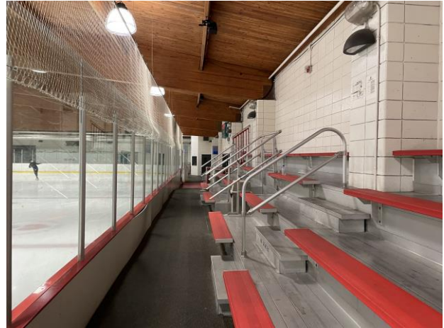
Photo 6 – Bleacher seating in ice arena
