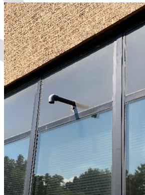
Condensation Drain out of window panel. No caulk around pipe / water & insect infiltration
