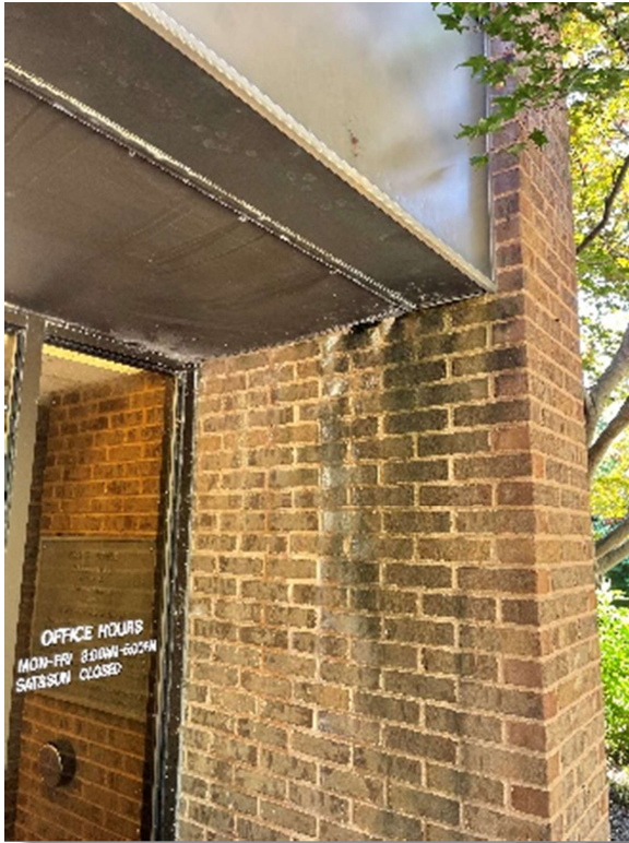
Water Damage to Canopy at City Hall Main Entrance
