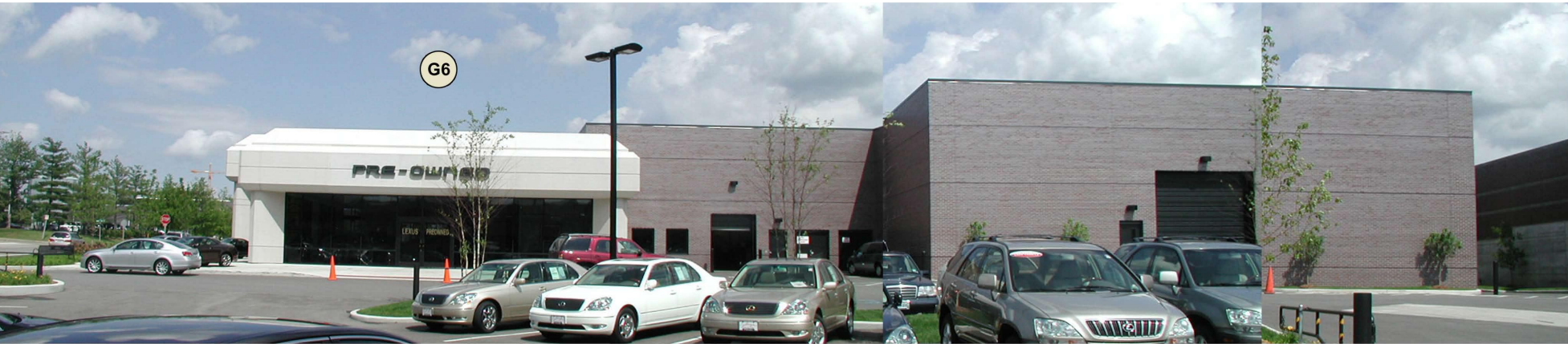
BUILDING 'G' - WEST ELEVATION
