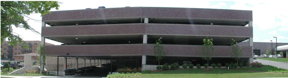
BUILDING 'H' - EAST ELEVATION
