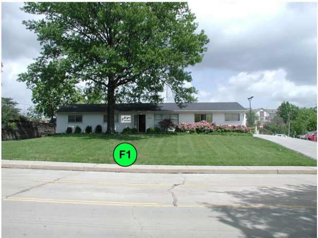
BUILDING 'F' - WEST ELEVATION
