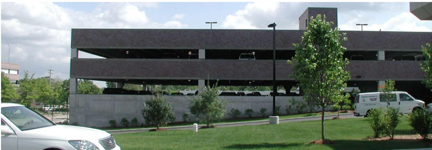
BUILDING 'H' - NORTH ELEVATION
