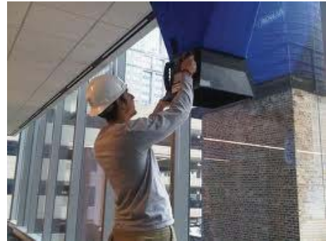
Photo 7 - Typical Air Balancing Activity
