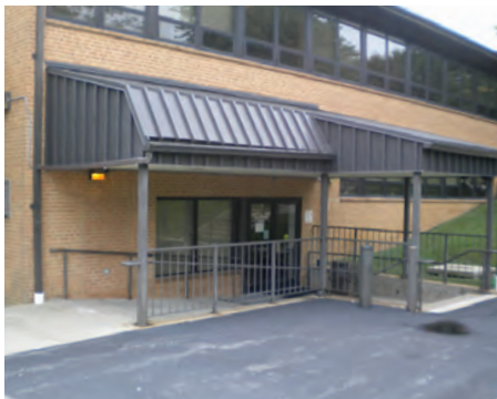
Enhance signage and wayfinding at Multi-Purpose entrance
