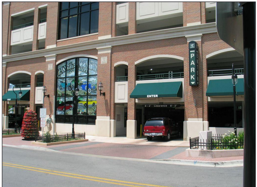
Figure 3: Parking garage (Naperville, IL)
