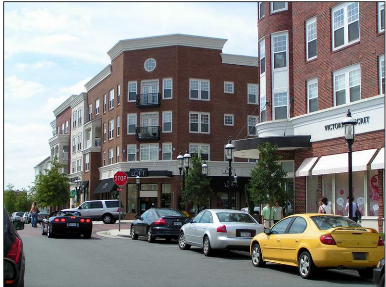
Figure 6: Brick is the primary material in these buildings with EIFS used only for banding and the facade change in the background (Birkdale Village – Huntersville, NC)
