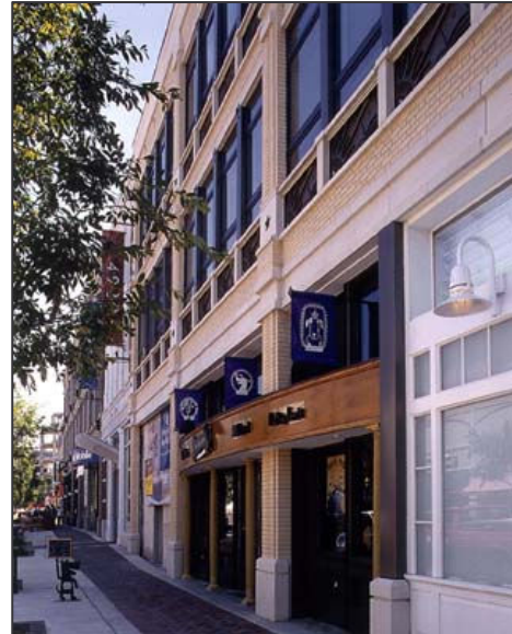
Figure 4: Recessed entrance and storefront windows (Bethesda Row, MD)
