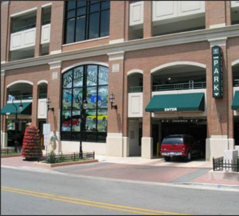
Mixed Use Parking Garage. High quality designed parking structures provide retail opportunities on ground floors and fit within the urban character of a traditional downtown.
