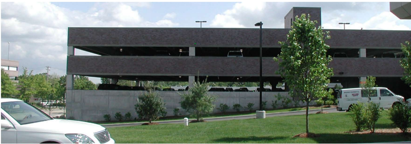
BUILDING 'H' - NORTH ELEVATION
