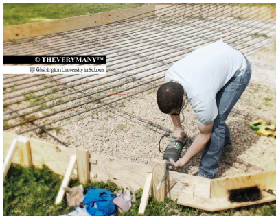
Formed Groundwork and Foundation
