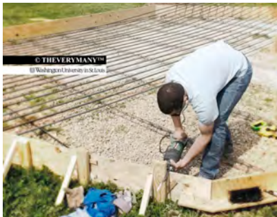
Formed Groundwork and Foundation
