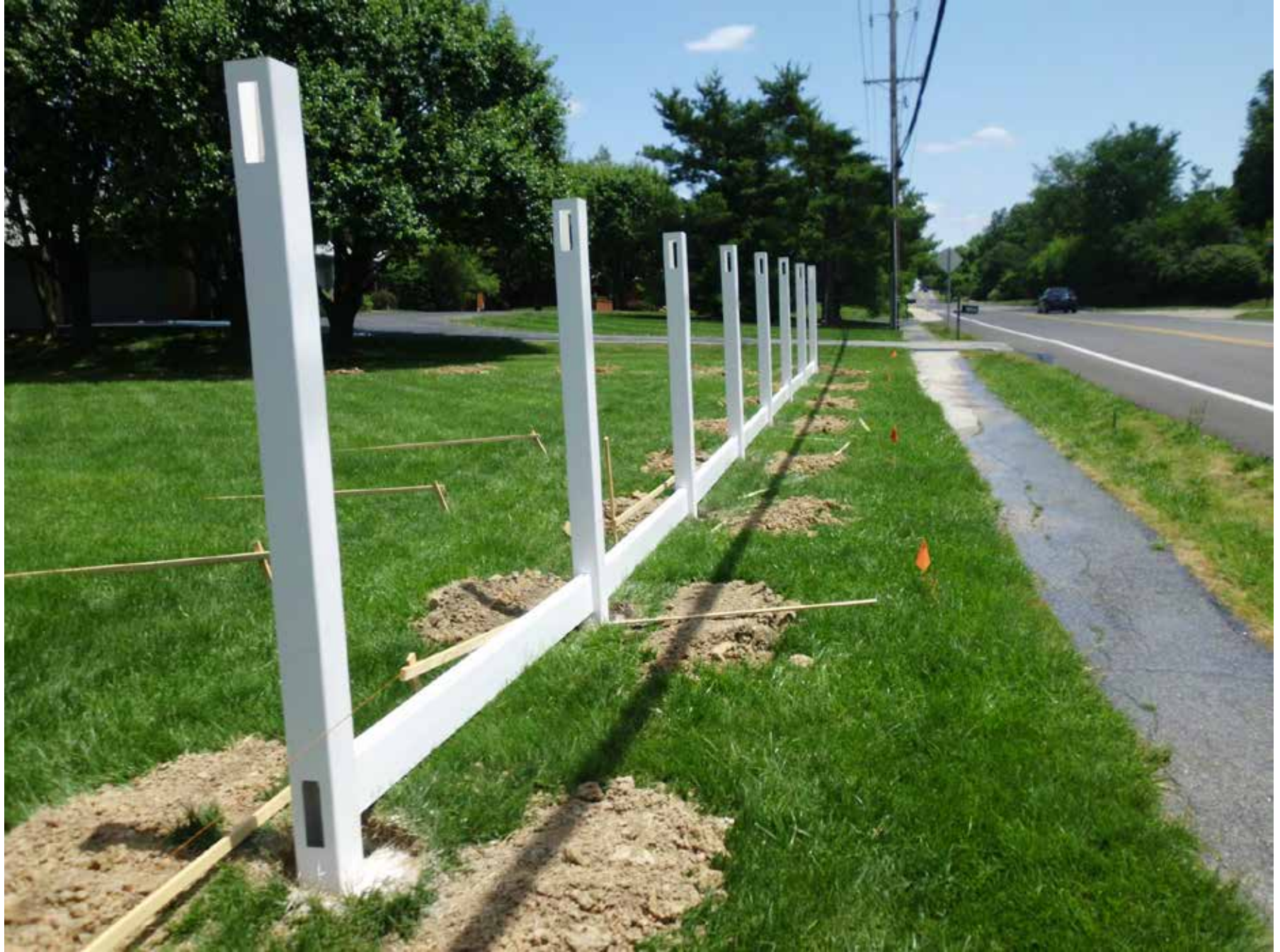
10 posts already installed in concrete
