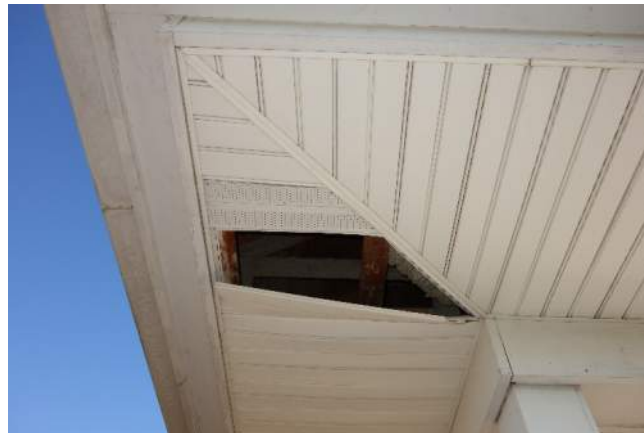
Figure 17 – Missing Soffit
