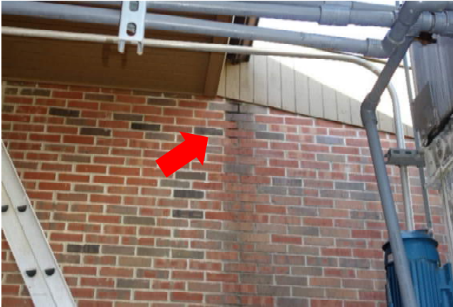
Figure 15 – Damaged Gutter Sections
