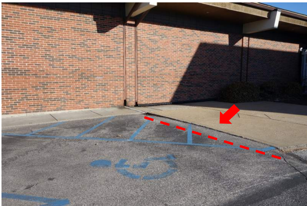
Figure 8 – Downspout Collection South wall of Ice Rink
