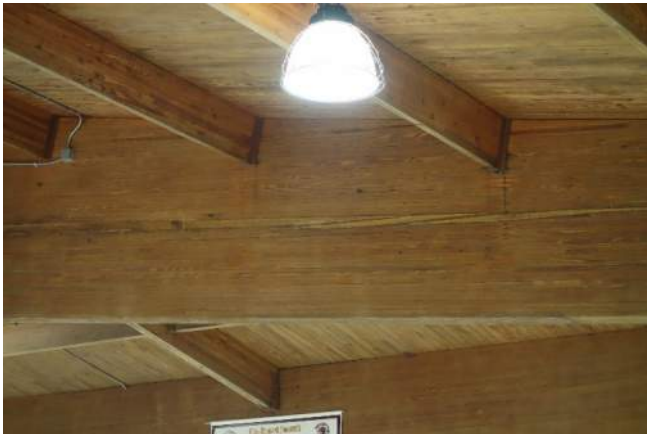
Figure 20 – Mass Timber Roof Beam
