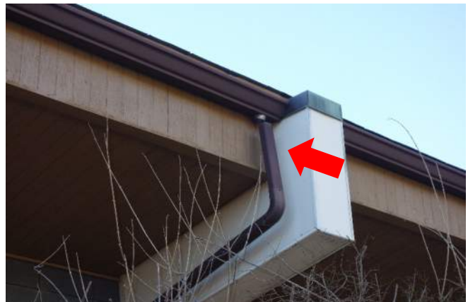
Figure 14 – Gutter Separation (North Side of ice Rink)
