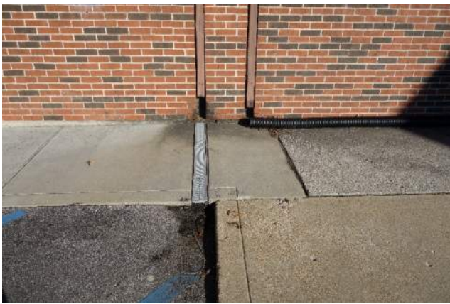
Figure 6 – Downspout Collection South wall of Ice Rink
