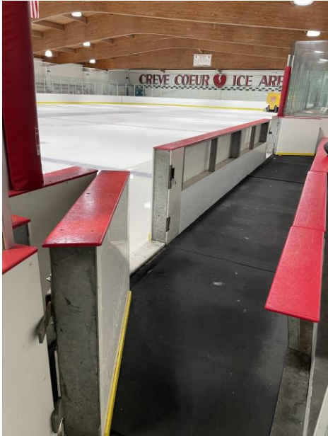
Photo 7 – Existing dasher board system
