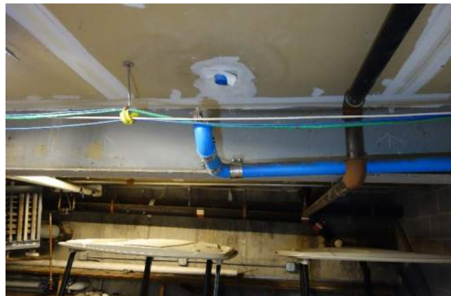
Figure 29 – Detached Pipe
