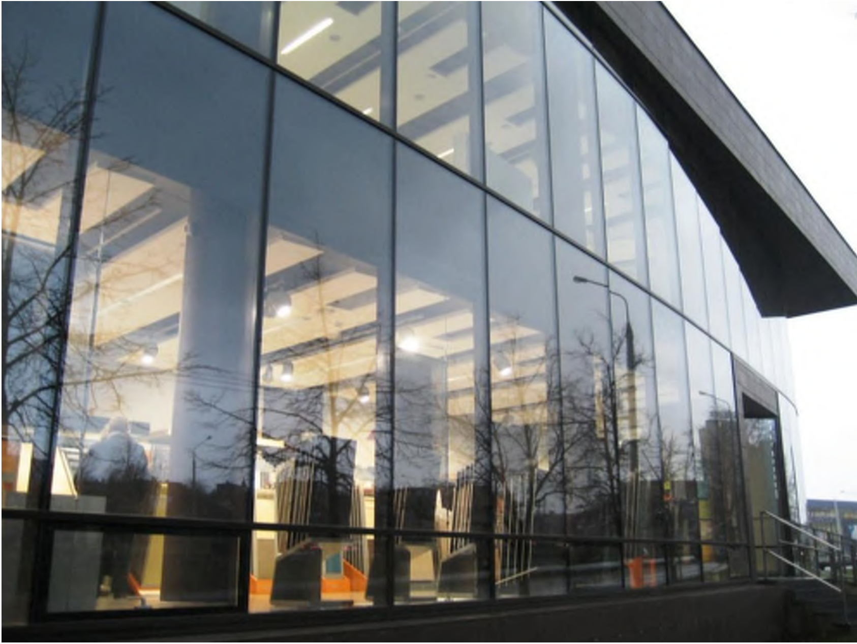
BUTT GLAZED CURTAIN WALL SYSTEM
