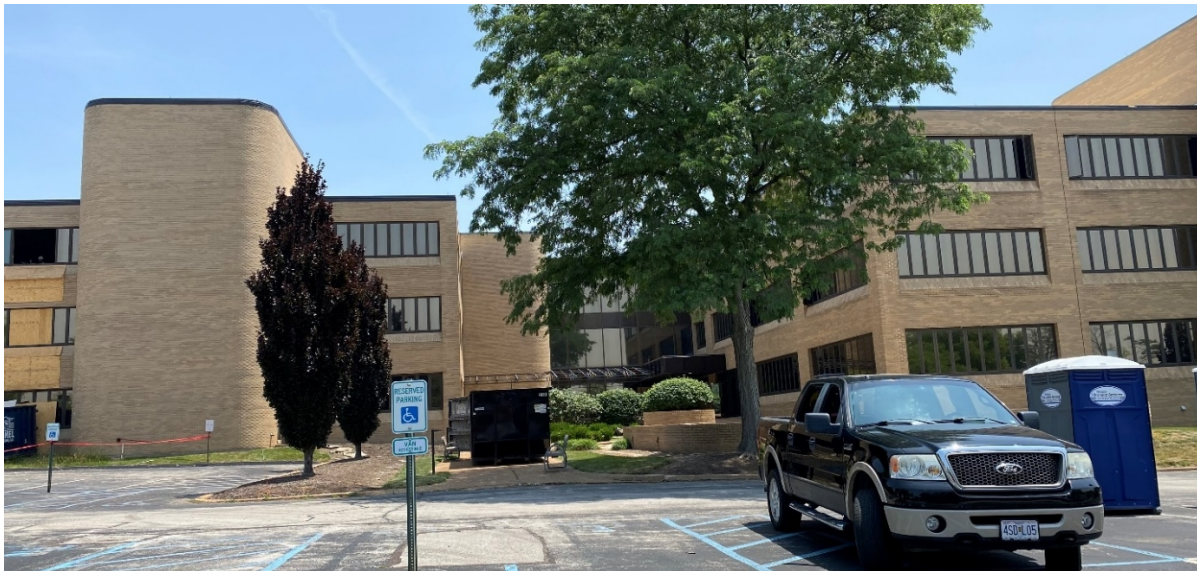
Figure 1: Existing façade of 717 Office Parkway
