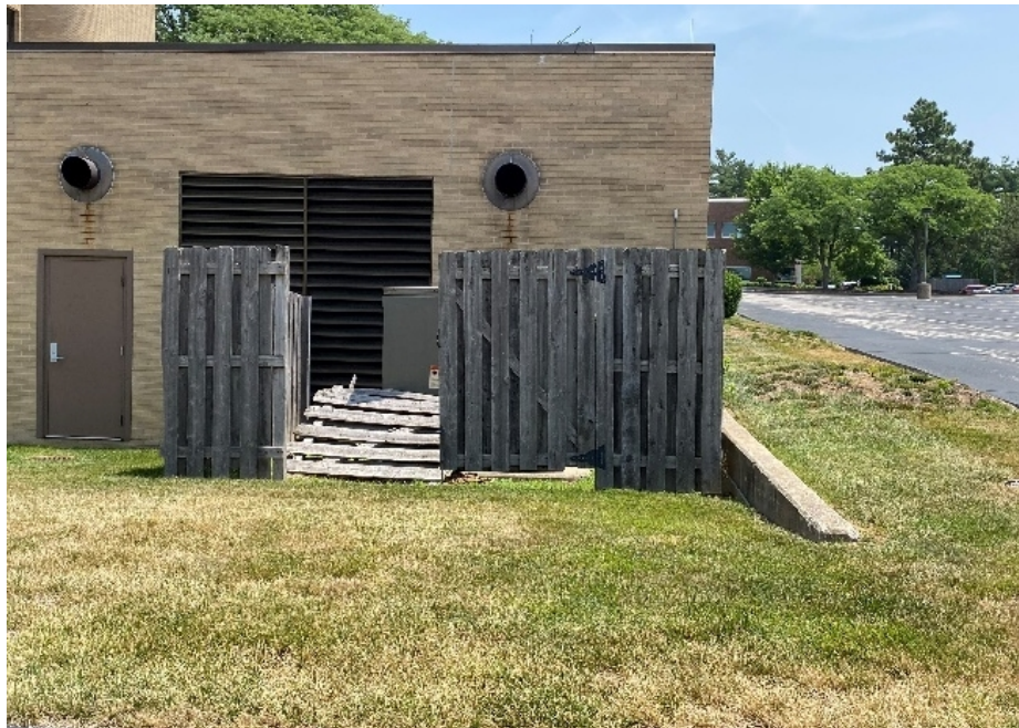
Figure 9: Existing utility enclosure.
