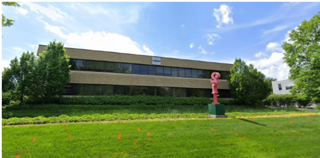
Figure 1: Existing façade of 211 N. Lindbergh Boulevard
