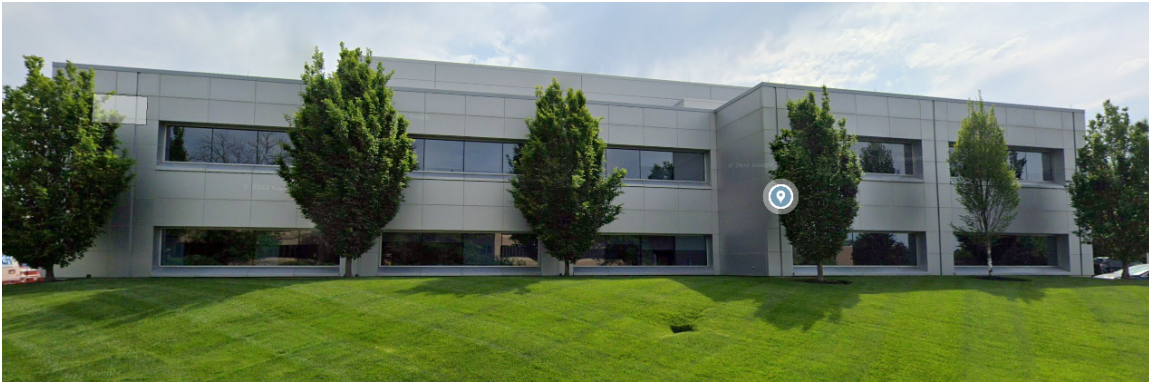
Figure 4: 744 Office Parkway directly across Office Parkway from the subject property.
