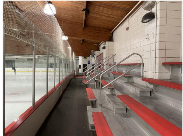
Photo 6 – Bleacher seating in ice arena
