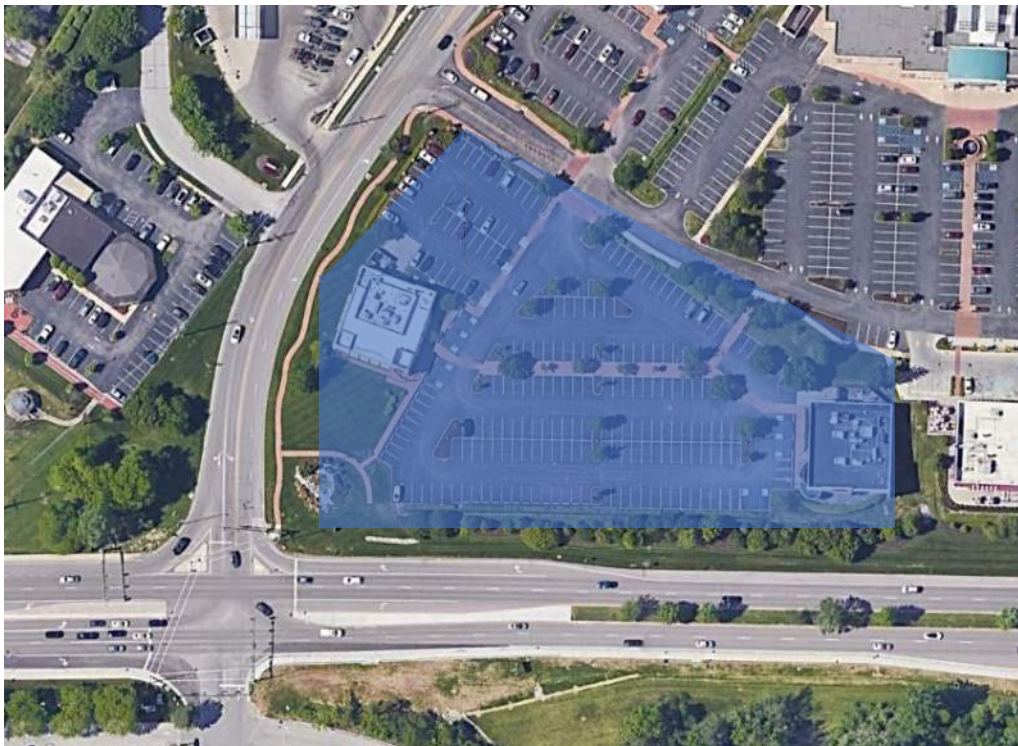
Figure 7 – Adjacent Altus Development
