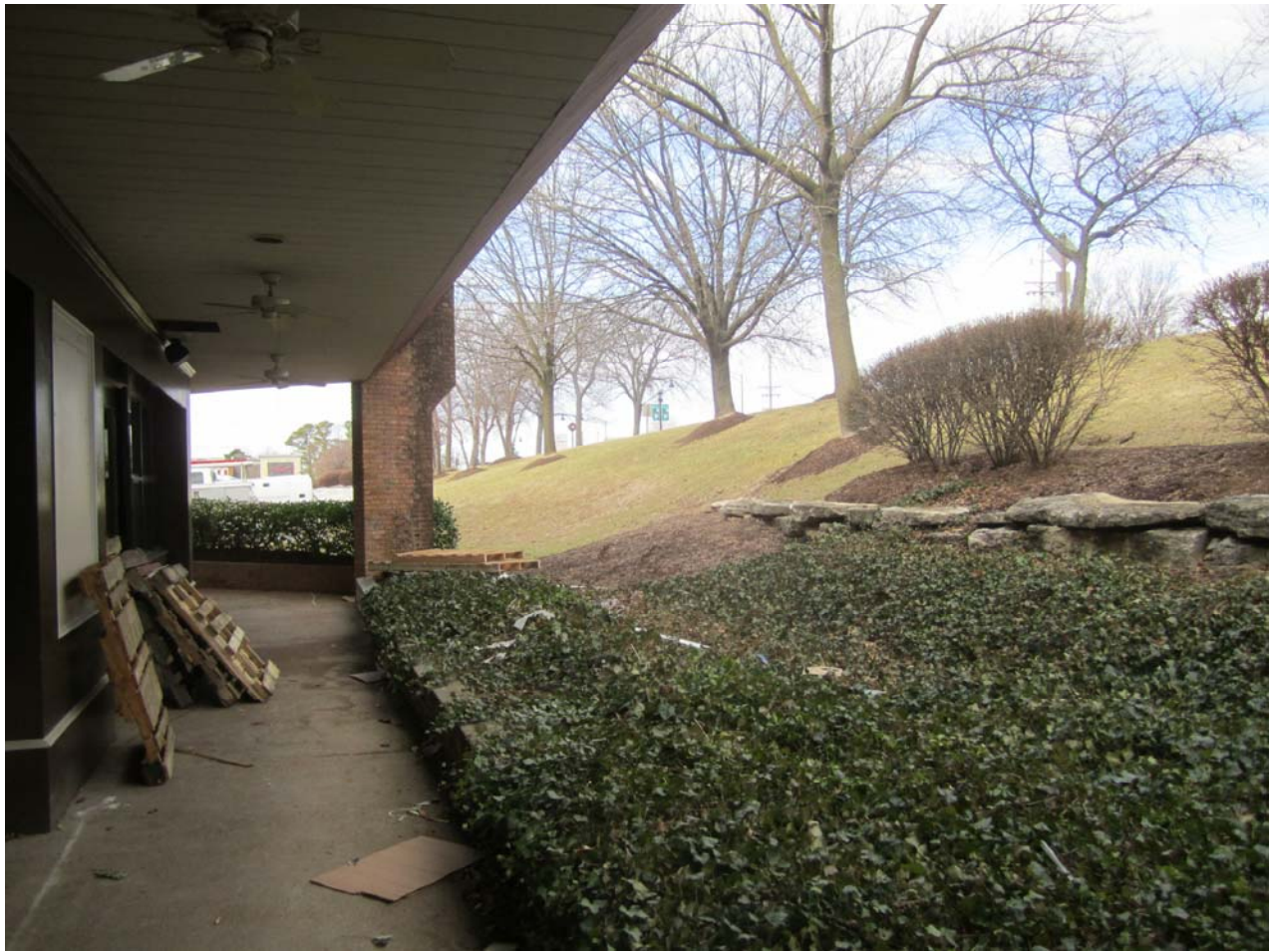
Existing Photo Looking West
