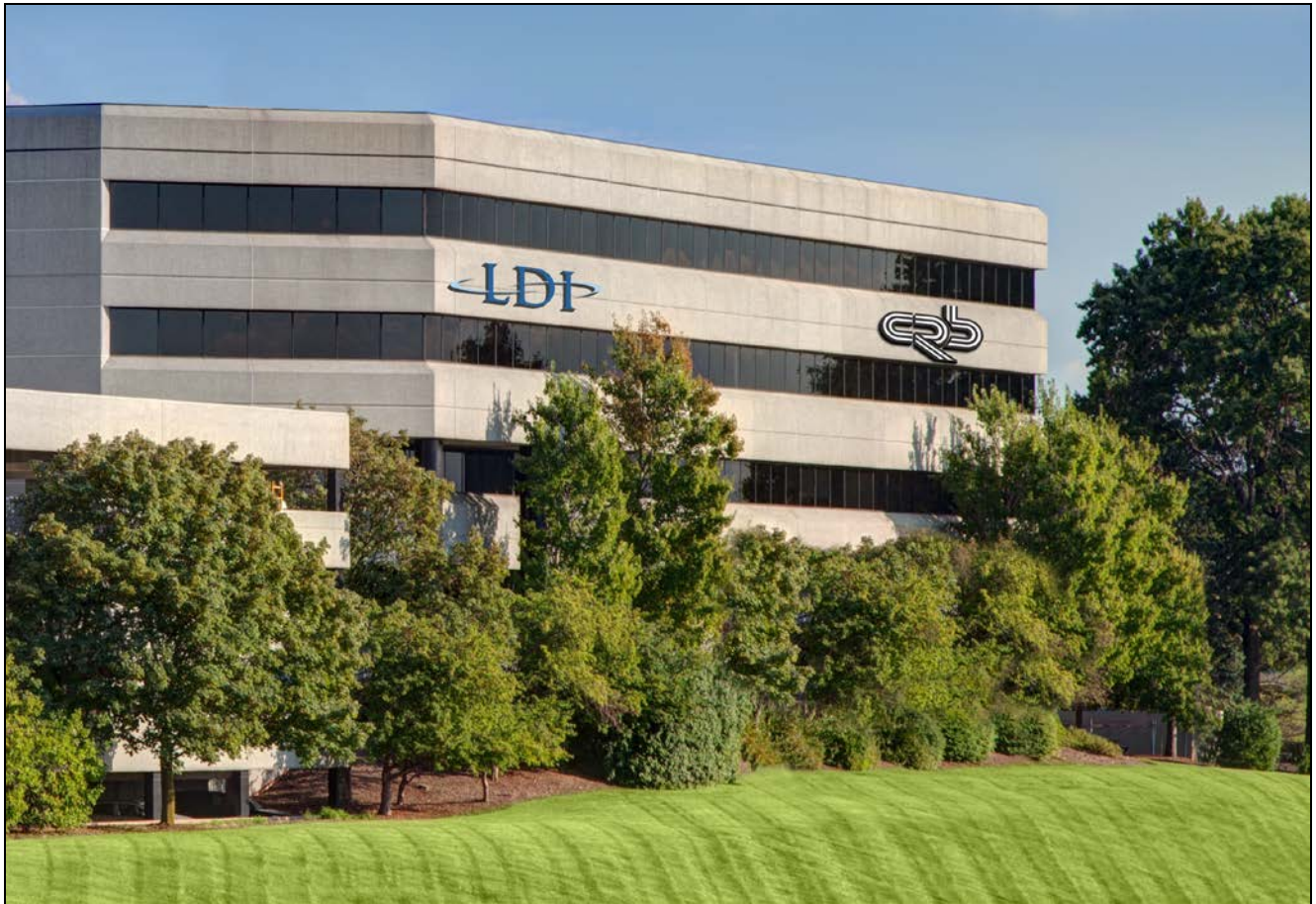
West facing elevation on North and South sides.
