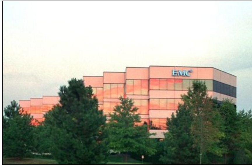
West facing elevation in the center.
