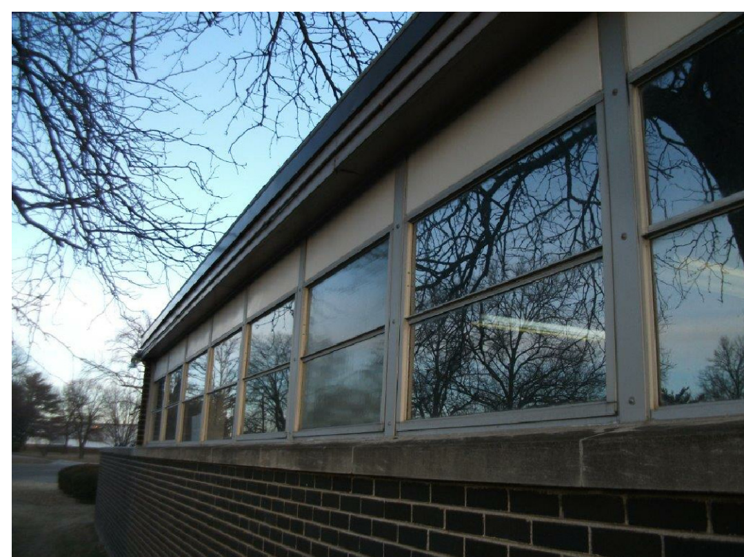
WEST ELEVATION LOOKING NORTH
