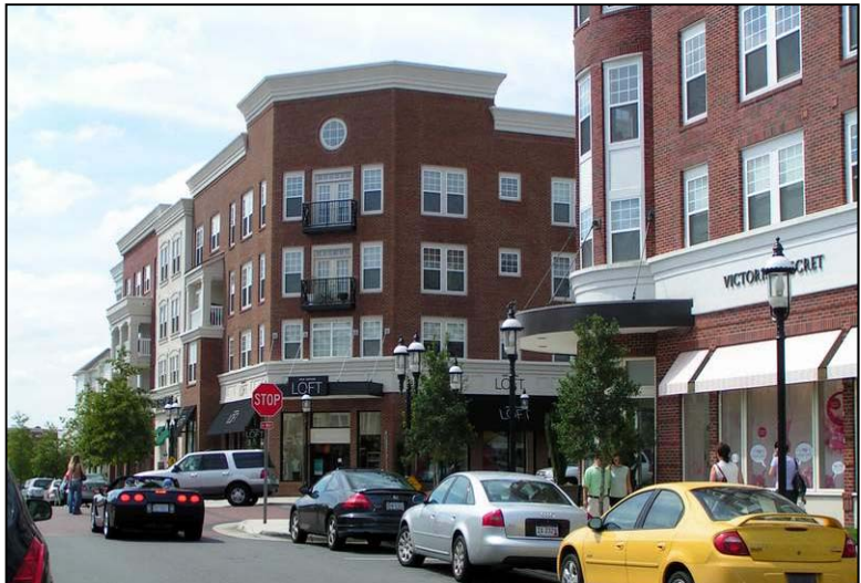
Figure 6: Brick is the primary material in these buildings with EIFS used only for banding and the facade change in the background (Birkdale Village – Huntersville, NC)
