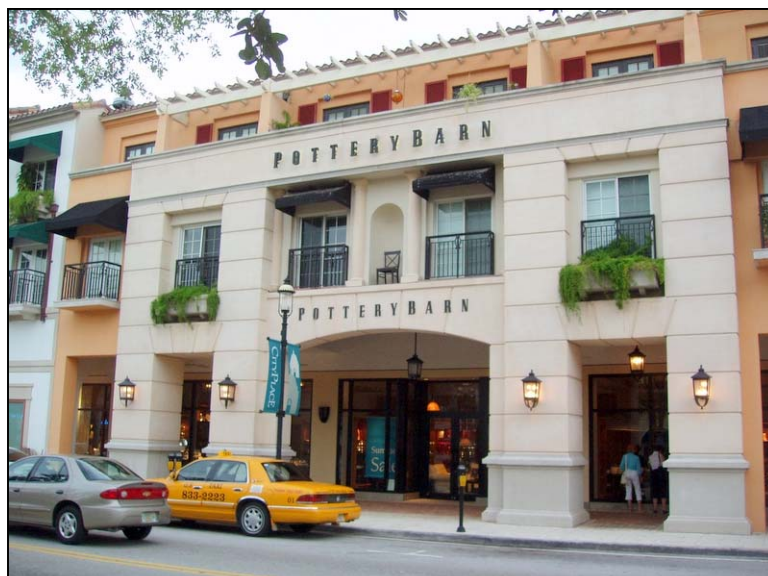
Figure 5: Recessed store entrance with an arcade or covered walkway (CityPlace - West Palm Beach, FL)
