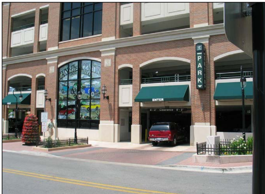
Figure 3: Parking garage (Naperville, IL)
