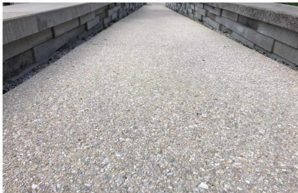
EXPOSED AGGREGATE SURFACES
