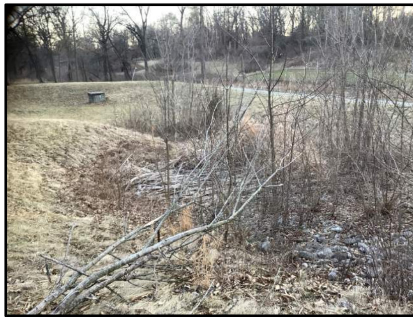
12. View west of Stormwater Feature 4- Constructed Basin.
