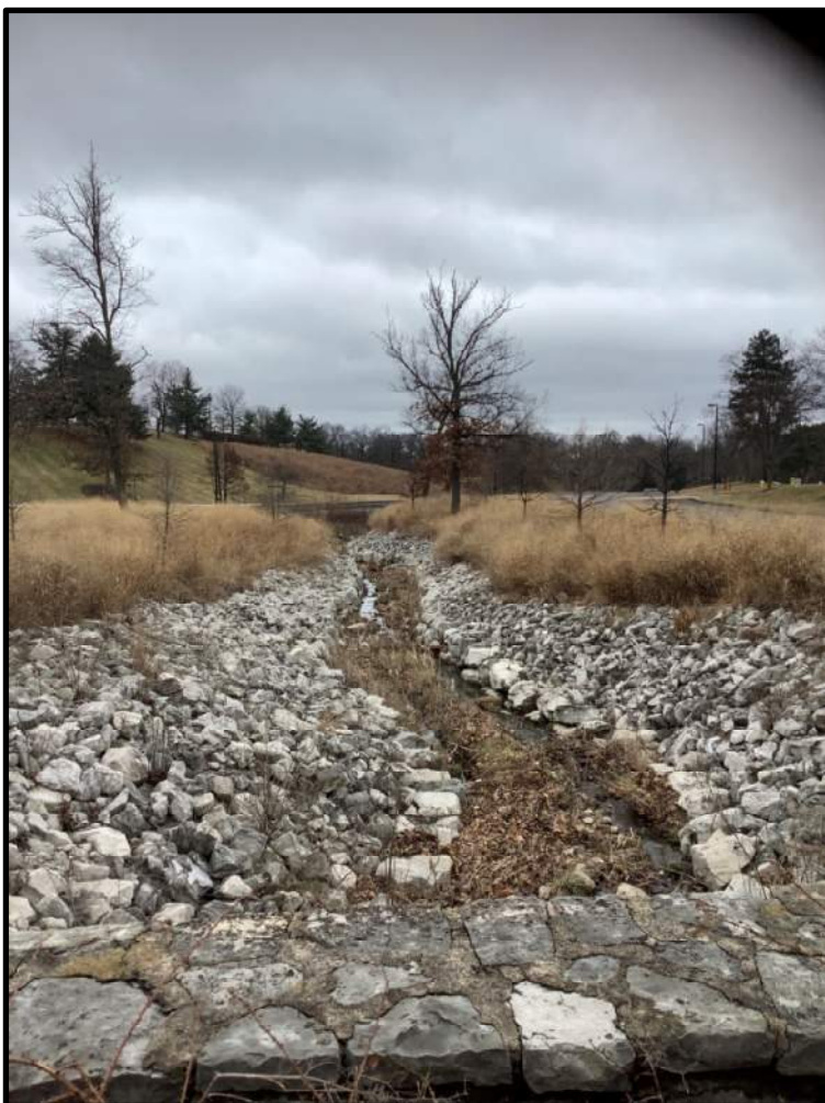
17. View south of Monsanto-Sunswept Creek, looking downstream at Reach 4.
