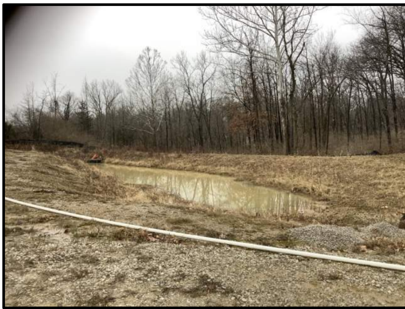
11. View southeast of Stormwater Feature 3- Constructed Basin.
