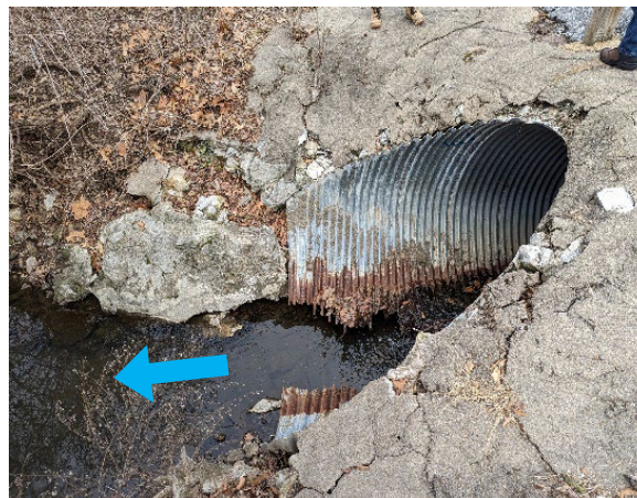
Photo of the downstream end of the culvert
