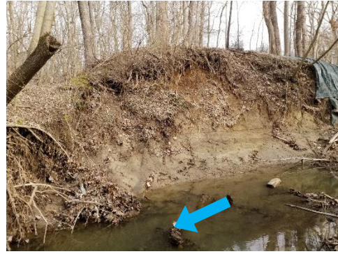
Figure 6-21: Outside bend erosion
