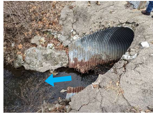
Figure 6-XX: Downstream end of culvert
