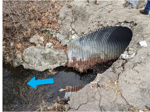
Downstream end of culvert
