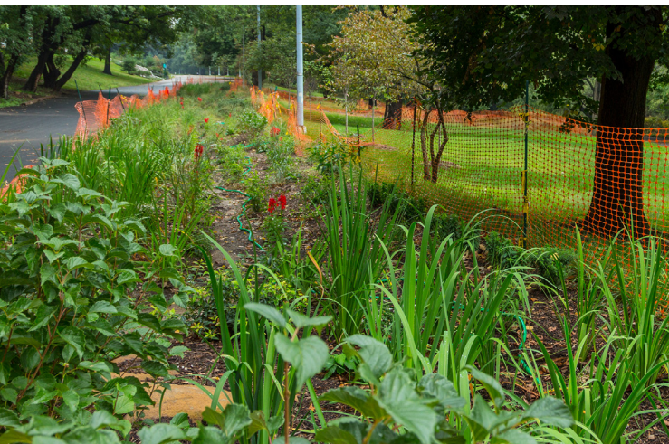
^ Figure 3. Green infrastructure, including bioswales and rain gardens can be an attractive way to reduce and infiltrate stormwater runoff from hard surfaces (image source: HDR)
