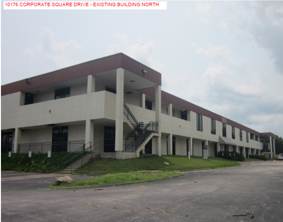
10176 CORPORATE SQUARE DRIVE - EXISTING BUILDING NORTH
