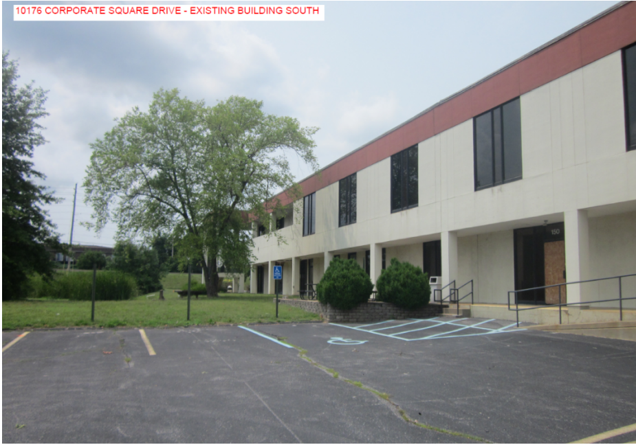
10176 CORPORATE SQUARE DRIVE - EXISTING BUILDING SOUTH
