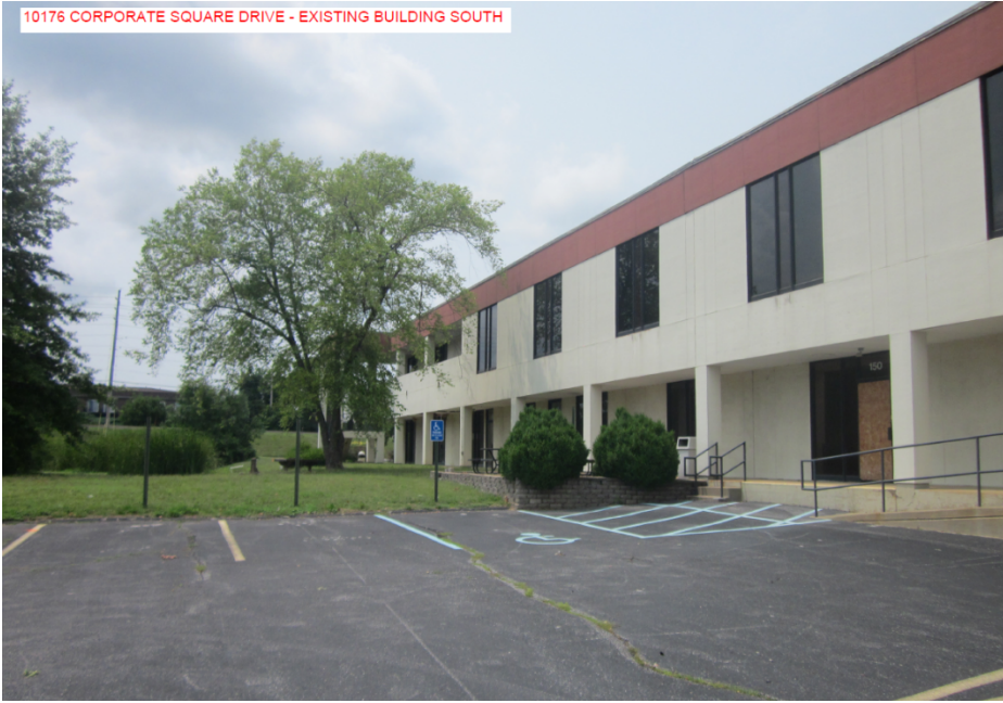
10176 CORPORATE SQUARE DRIVE - EXISTING BUILDING SOUTH
