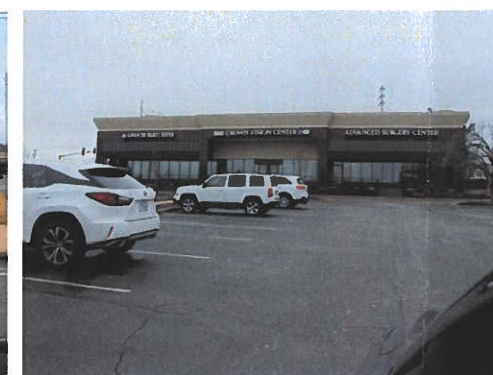
12601 (NORTH ELEV.) TENANT WALL SIGNS
