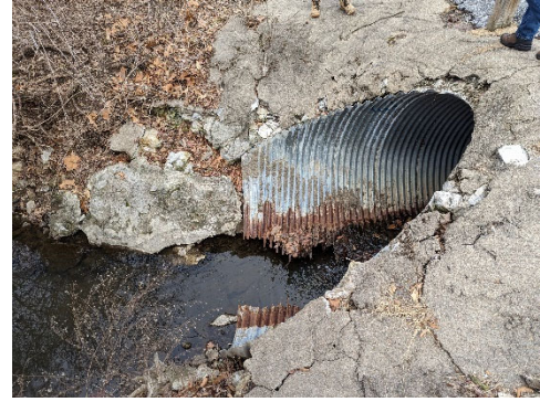
Downstream end of culvert
