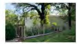
Utilities Example (Storage Tank)
