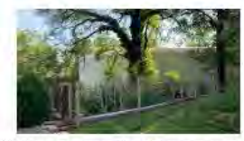
Utilities Example (Storage Tank)
