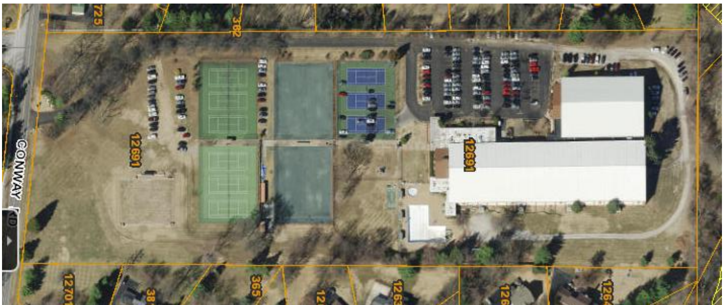
Figure 1: 2014 St. Louis County Aerial Photo of Parking Issues on Site.
