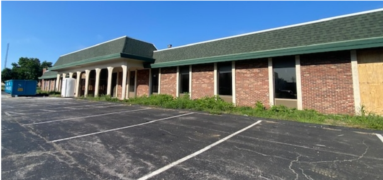
Figure 1: Existing façade of 1260 Andes Blvd.
