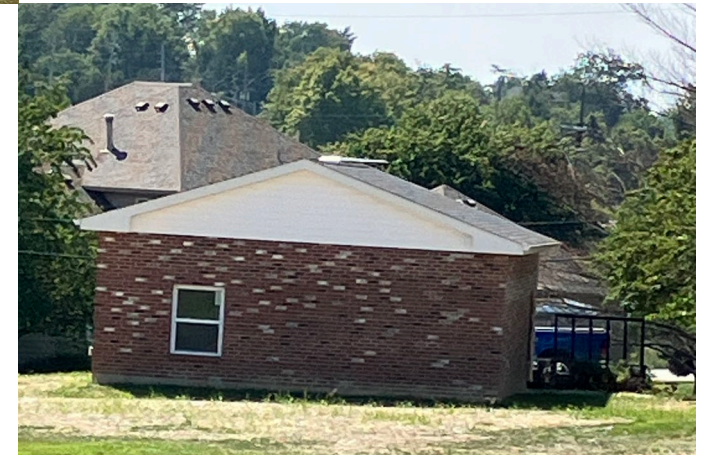
New Accessory Structure
