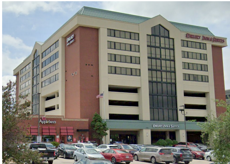
Figure 2: Existing Front/North Elevation.
