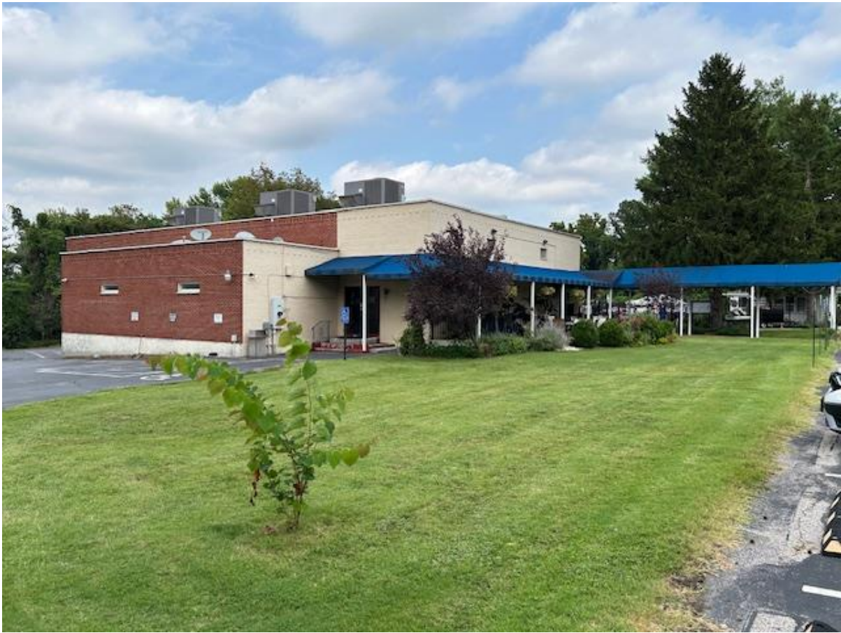
Lodge Hall Building – South Face
