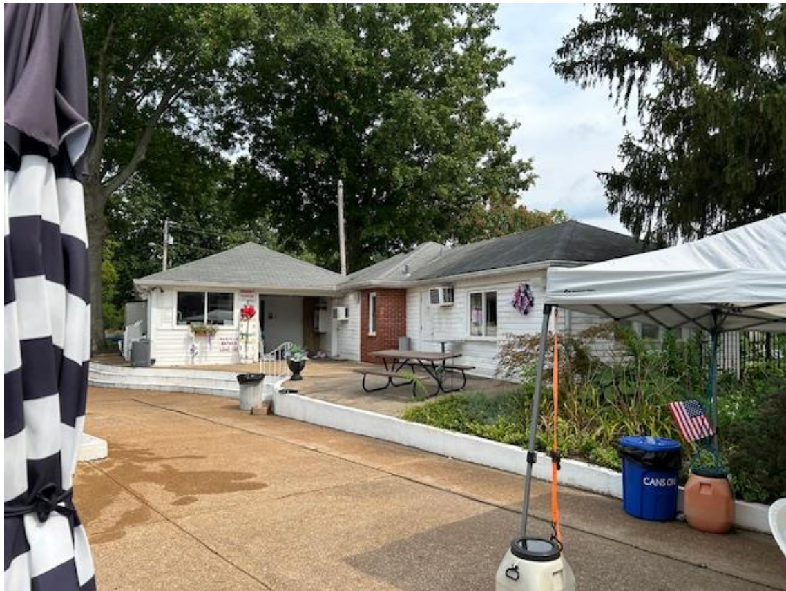
Bathhouse Office Complex – North Face
