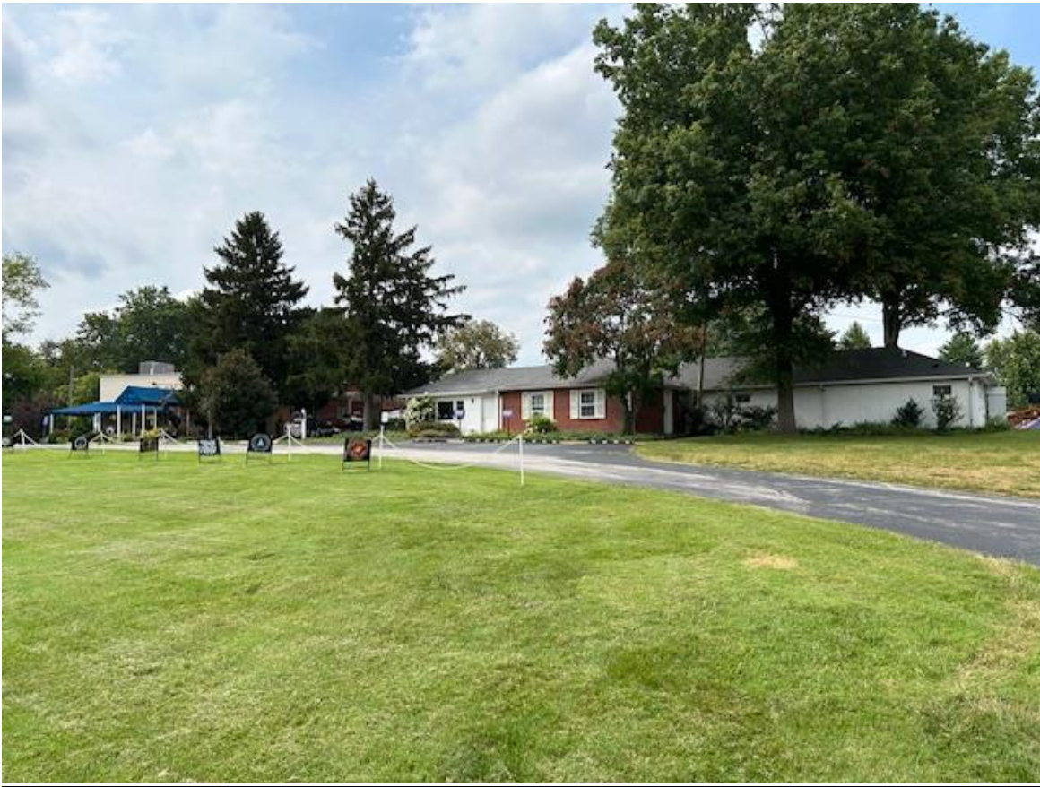
Bathhouse Office Complex – South Face
