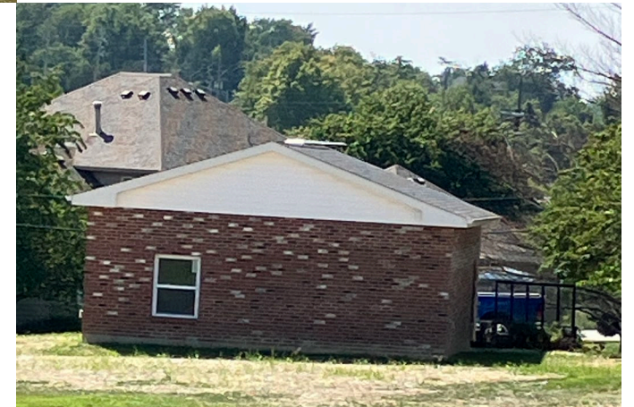
New Accessory Structure
