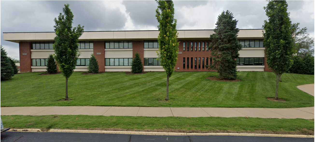
Figure 2: Existing Administrative Building.
