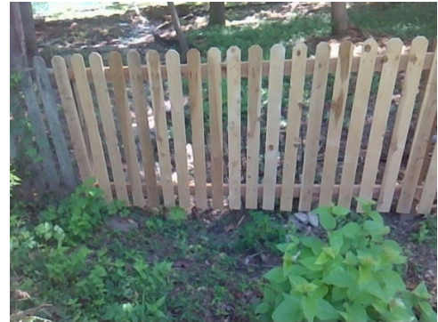
West side of fence
