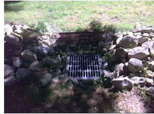
Existing yard drain on west property line of #8
