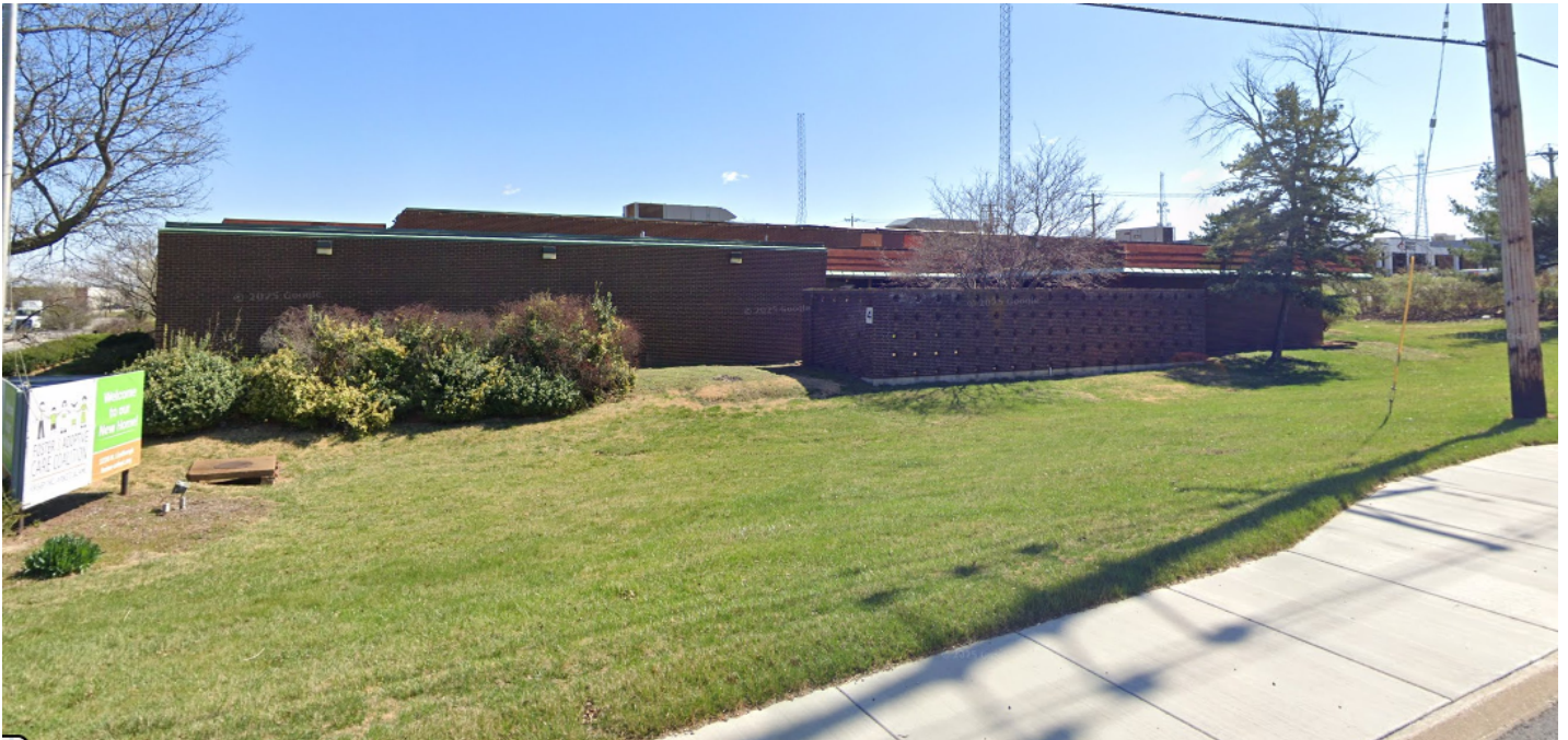
Figure 2: Existing façade of 1220 N. Lindbergh from March 2025 Google Street view taken from N. Lindbergh.
