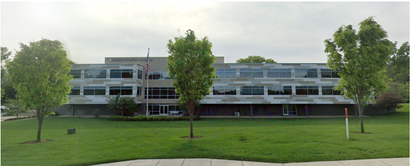
Figure 7: Façade Alterations at 243 N. Lindbergh Blvd approved in June 2015 by Site Development Plan.
