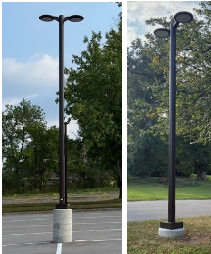
Figure 1. Existing light poles installed in 2024 on varying sized bases.
