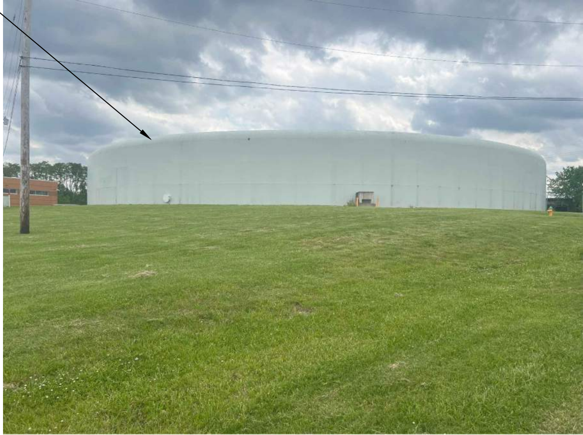
TANK NO. 2 PHOTO 1
