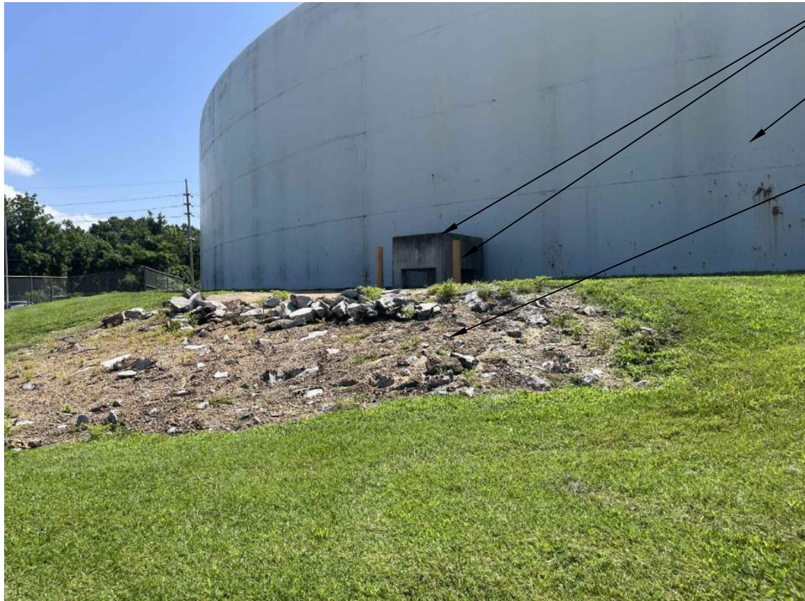
TANK NO. 2 PHOTO 2
