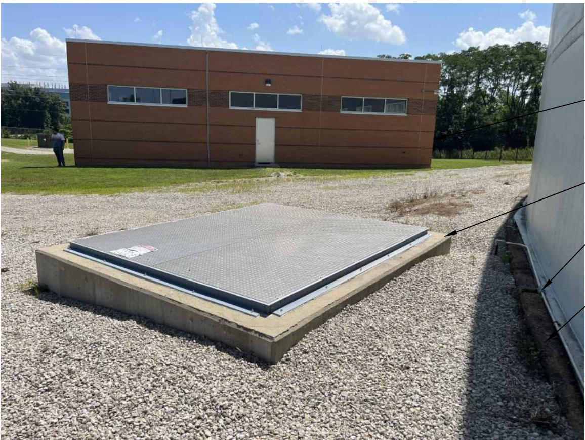
TANK NO. 2 VAULT PHOTO NO. 1
