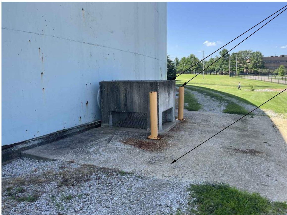
TANK NO. 2 PHOTO 3
