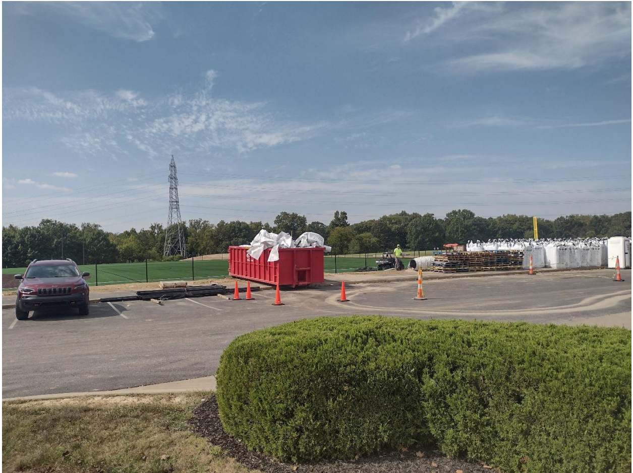
Looking West from proposed tower location
