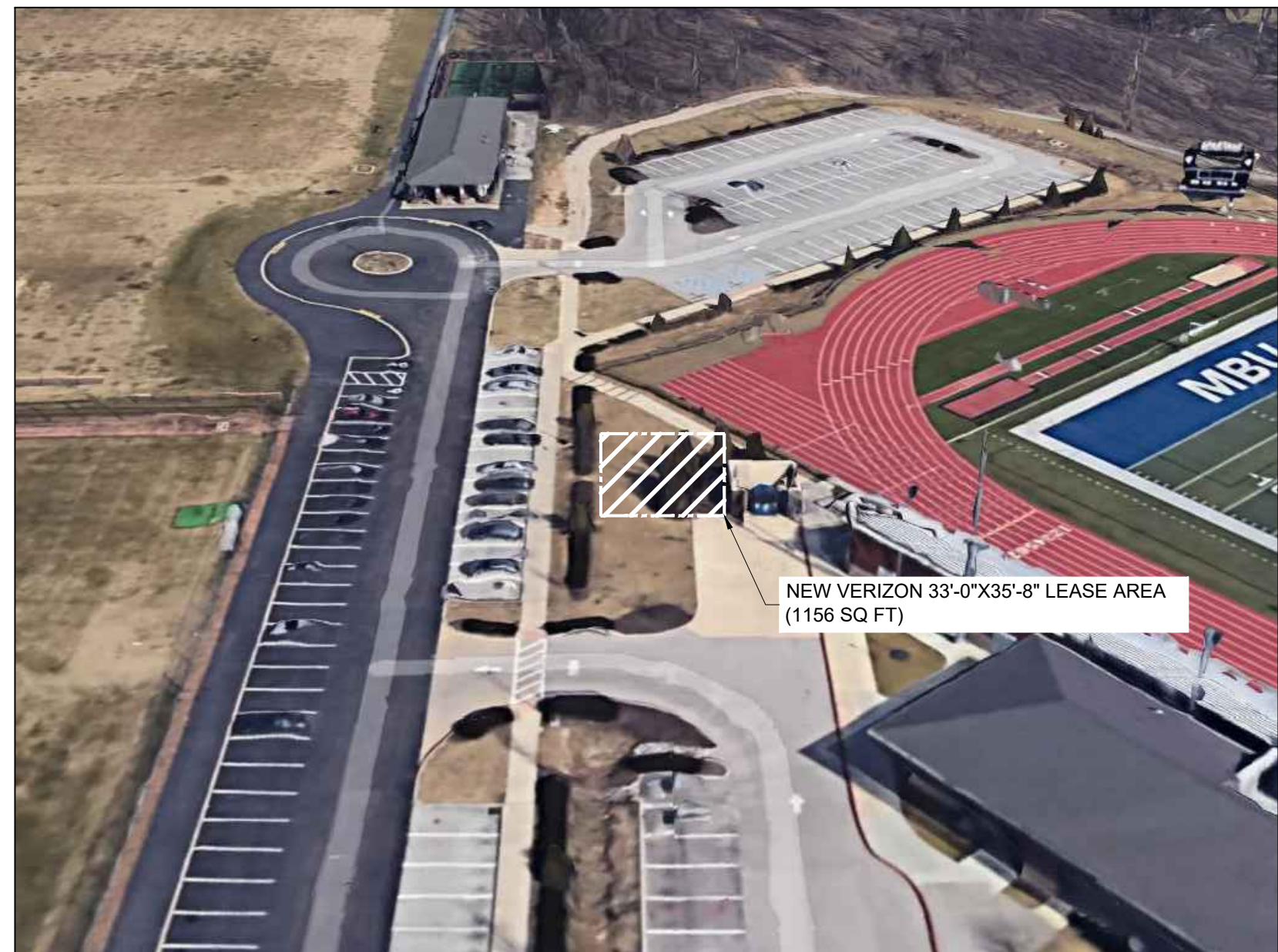
VIEW OF NEW LEASE AREA (LOOKING NORTH)
