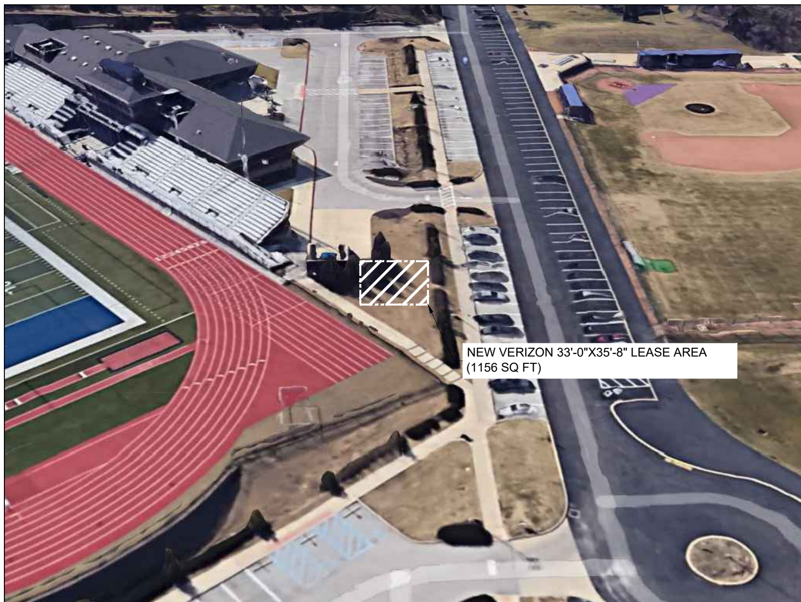
VIEW OF NEW LEASE AREA (LOOKING SOUTH)
