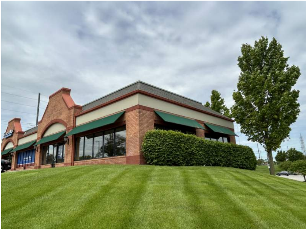
4 EXISTING SITE PHOTO
