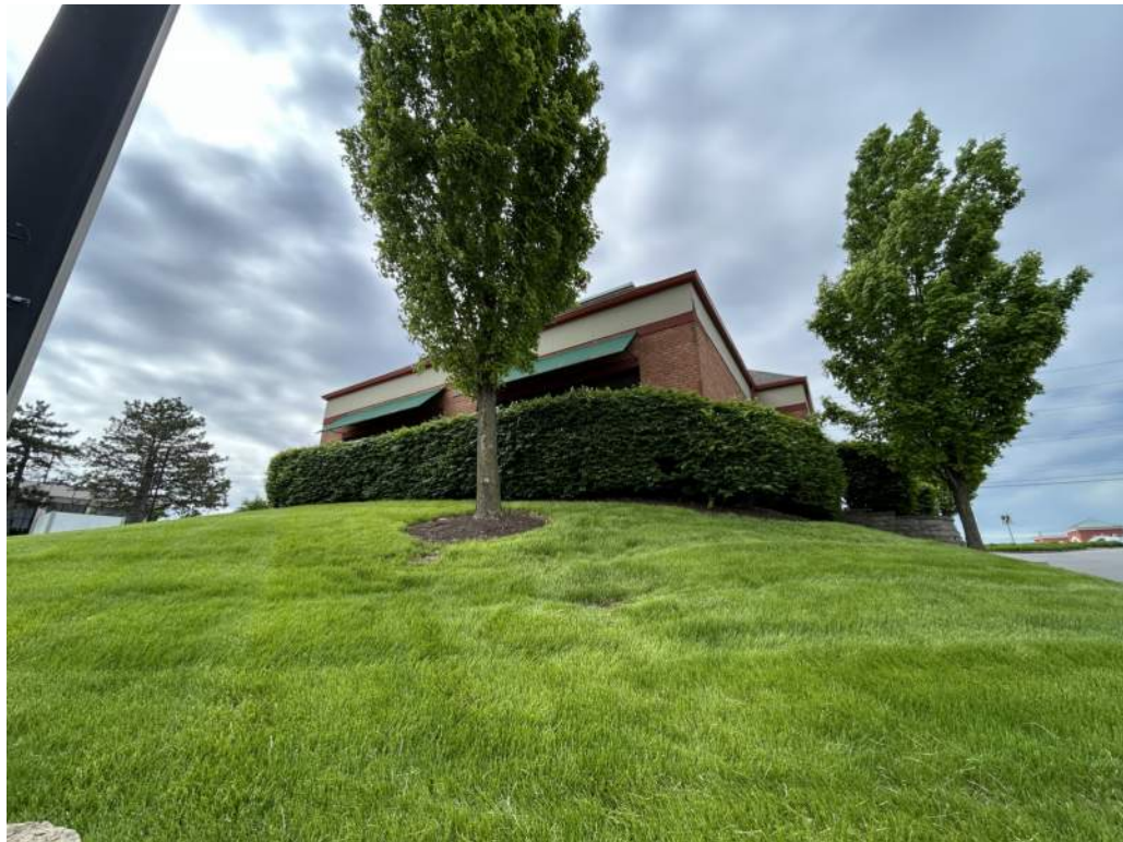
6 EXISTING SITE PHOTO
