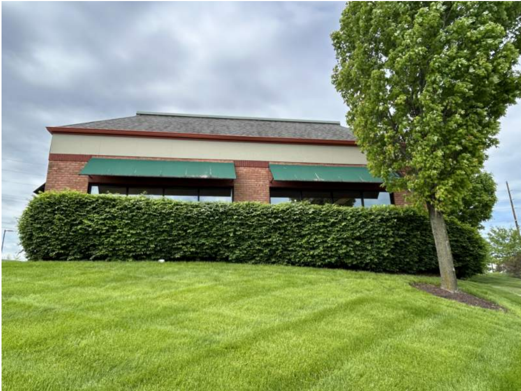
5 EXISTING SITE PHOTO
