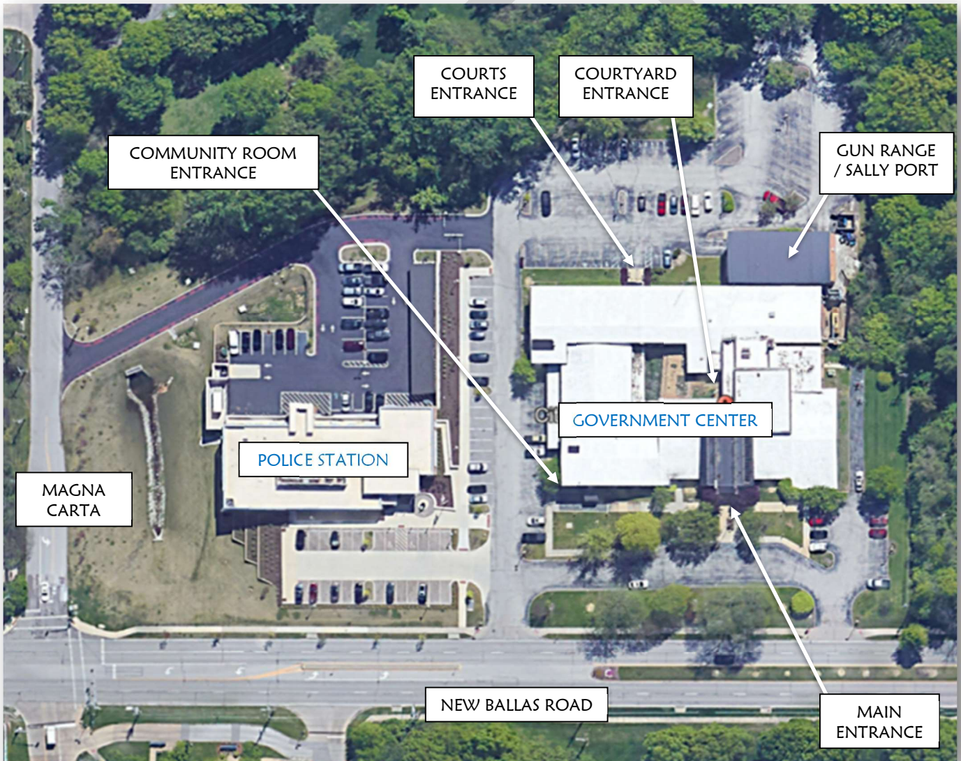
Enlarged Aerial Photo from Google Earth displaying feature elements at the Government Center Property.
