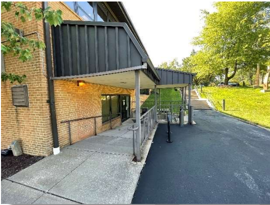
Entrance to Community Room at Northwest Corner of Building
