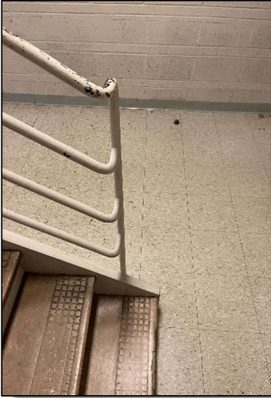
View of horizontal guardrails and shortened rail extensions.
