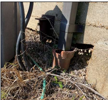
Photo showing foundation support of breakroom floor
