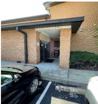
Entrance to Gymnasium on Northwest corner of Building.
