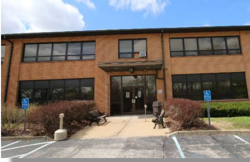
Exterior of East Entrance
