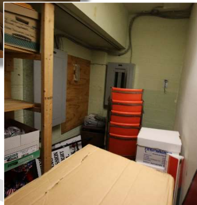
Electrical closet has been utilized as storage and now electrical panels cannot be accessed resulting in code violations.
