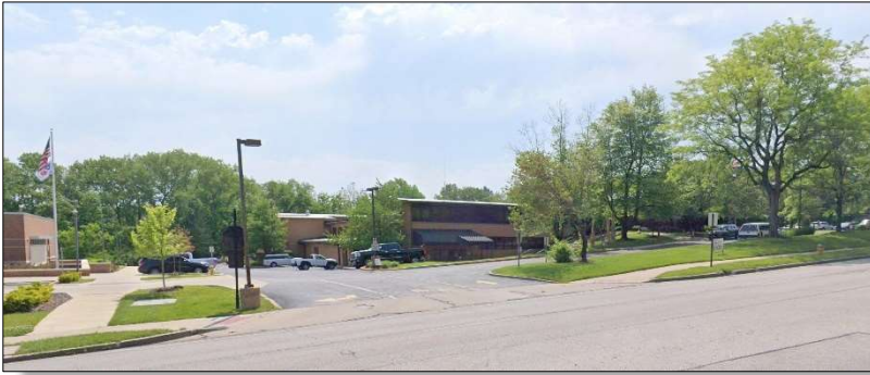
View of Existing Main Entrance Lobby / Skylights along South side of Lobby
