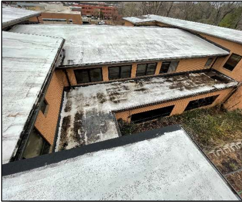
Example view of existing roof condition overlooking lower hallway and Gym.
