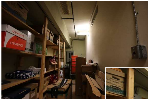
Electrical closet has been utilized as storage and now electrical panels cannot be accessed resulting in code violations.
