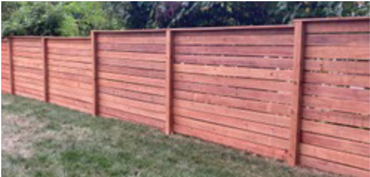
Figure 2: Fence detail showing 6-foot-tall horizontal, wooden, privacy fence.
