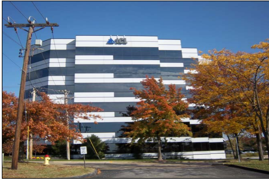
West facing elevation in the center.
