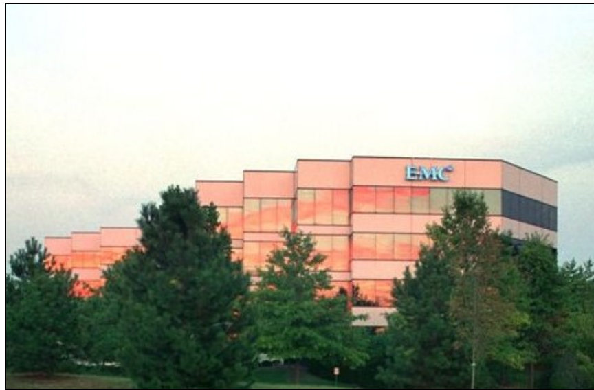
West facing elevation in the center.
