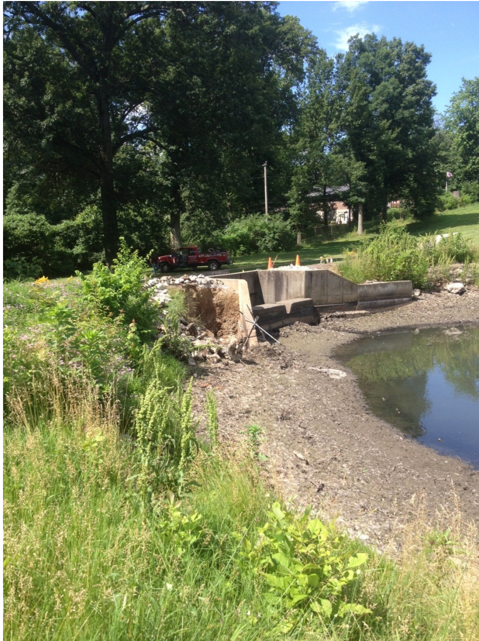
Photo 2: A view of the dam and spillway during the repair of the first breach. Note that the lake was drained an additional foot to reduce flow through the breach and the additional erosion that would cause.
