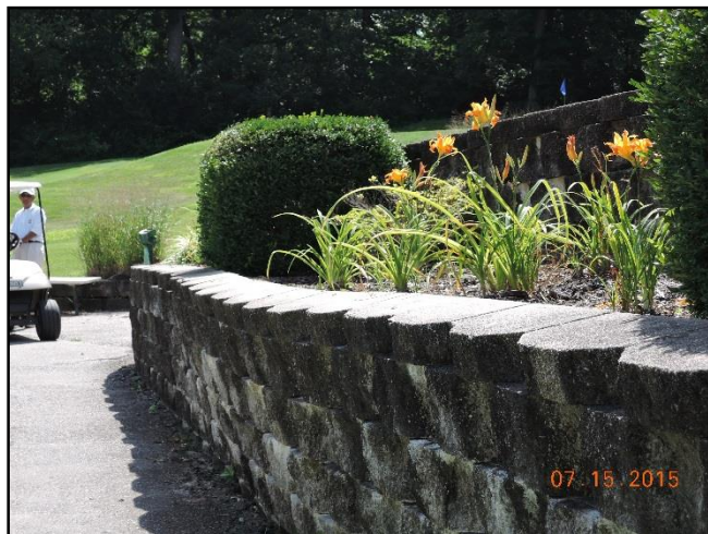
Photo 10 retaining wall at 4 tee
