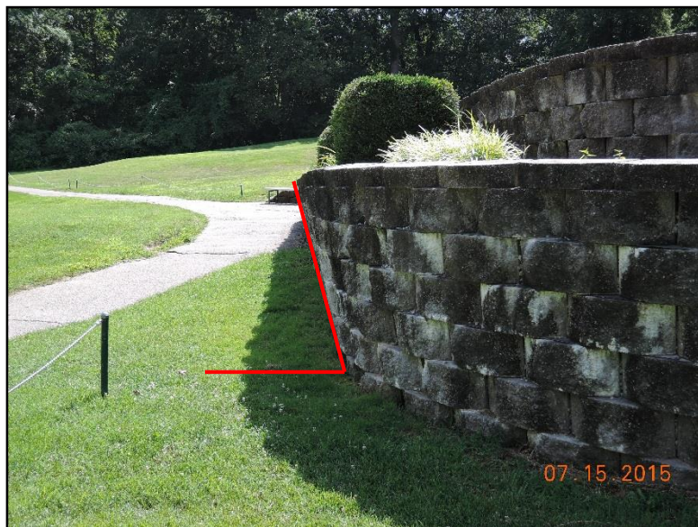
Photo 4 Retaining wall at 4 tee
