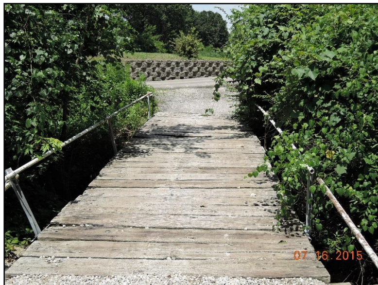
Photo 15 Equipment bridge at number 5
