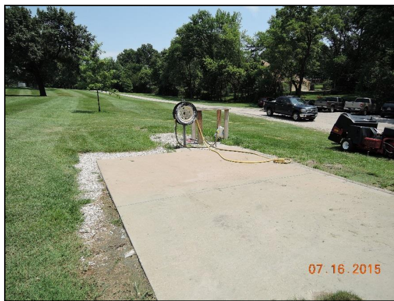
Photo 3 Wash pad at maintenance facility
