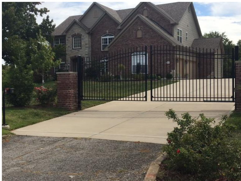
Figure 4: Home at 12068 Ladue Road, columns and gate were permitted, but a fence was not, so the property owner planted a hedge.
