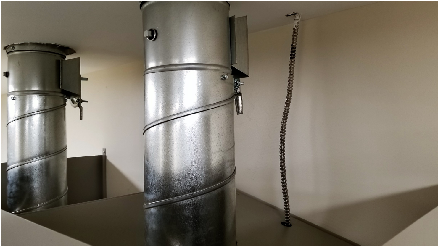
Example of HVAC connection and Power Feed connection. Hole in sloped tops to be done by HVAC and Electrical contractor.
