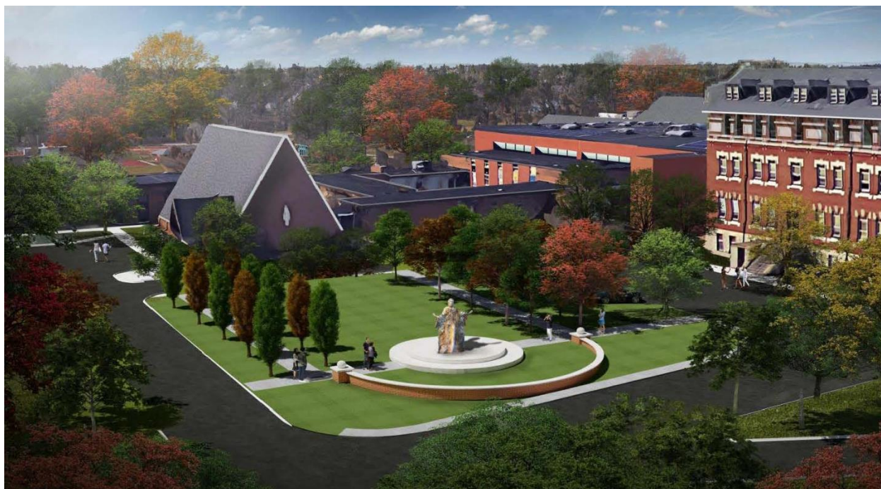
Figure 9: Close-up of a future sculpture and garden area
