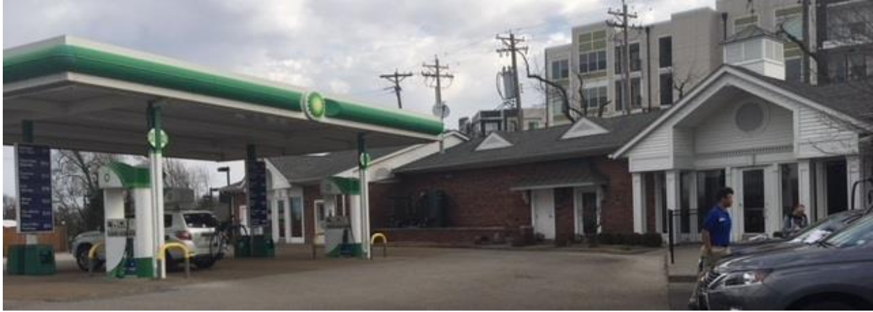
Figure 6: Photo of Existing Building and Canopy Structure
