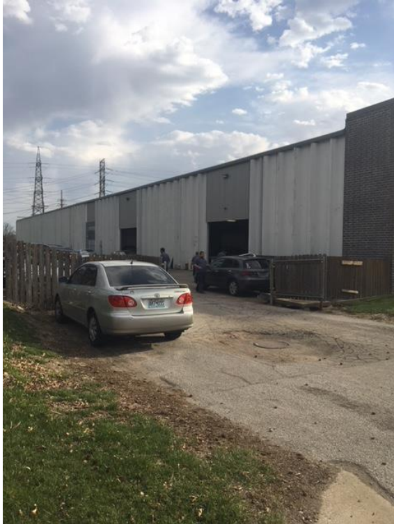
Figure 2: Photo of the existing fenced area on the west side of the building.
