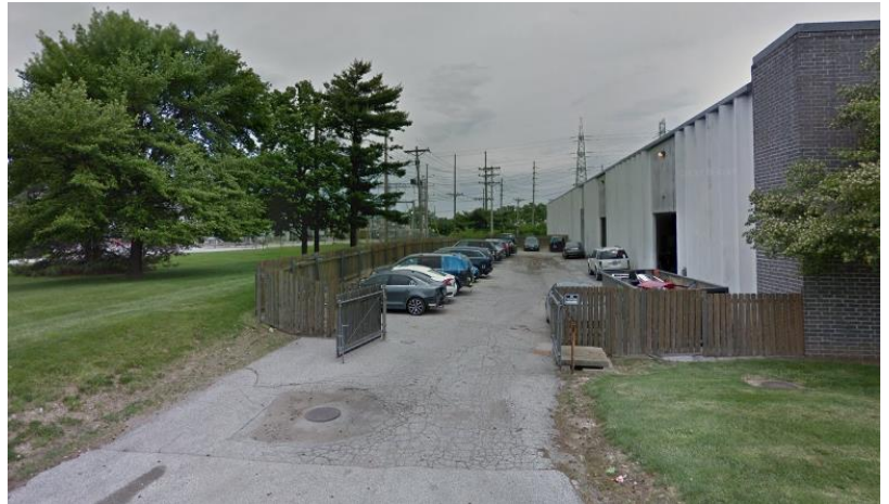
Figure 3: google Image of the fence area on the west side of the building.
